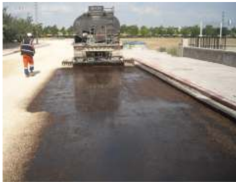
Terrapime with Cationic Bitumen Emulsion
